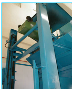
Binlifter designed to lift 2 X 240 ltr OR 1 X 660 ltr DIN bins.
