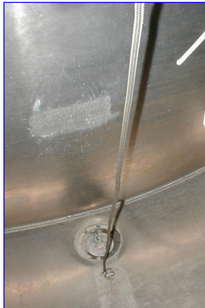
Anti-static > 32 mm diameter INOX cable (Applicable for Exxon tank only)
